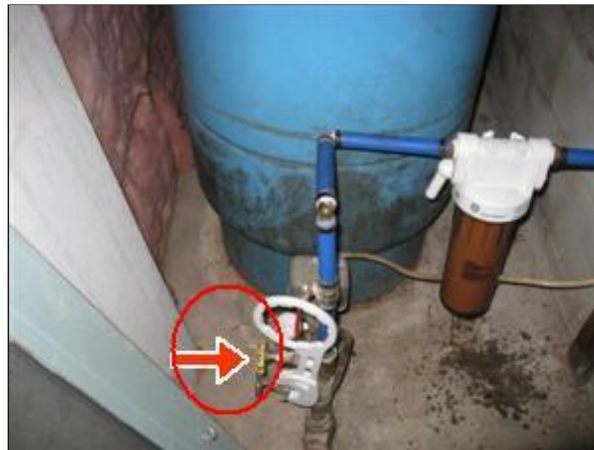
4.3 Picture 1 In basement
