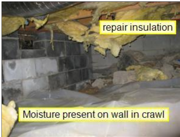
1.0 Picture 1 crawlspace under kitchen
