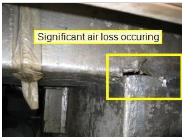
6.3 Picture 1 crawlspace new addition
