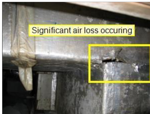
6.3 Picture 1 crawlspace new addition
