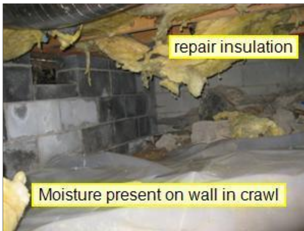
1.0 Picture 1 crawlspace under kitchen
